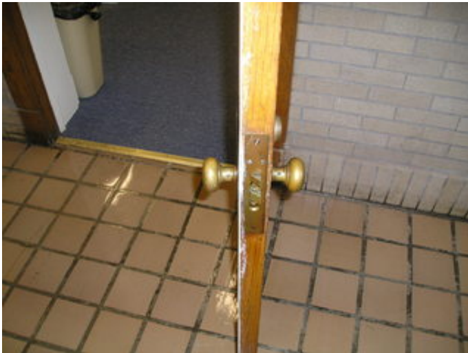
Replace with lever type hardware
