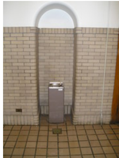
Non-accessible drinking fountain in original 1922 building.
